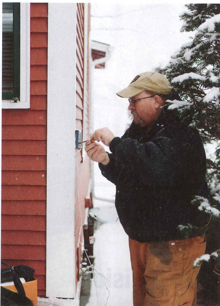
Operator Michael Coyle works on installing a new meter at a customer's home. A new automated metering system (Zenner USA) enables staff to read meters remotely.
