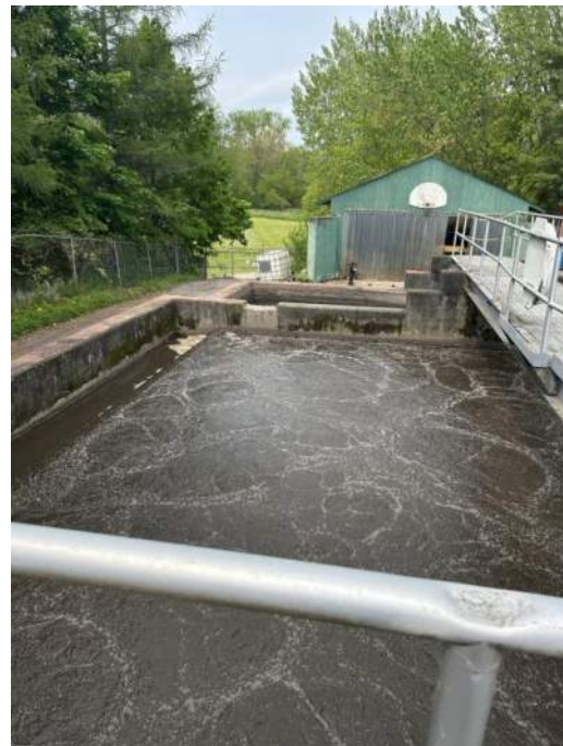
Figure 2-14 Biological Aeration Tank
