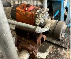
**Floccualtor:** The flocculator seal shaft has been leaking for some time. It's hard to tell the extent of the damage.
