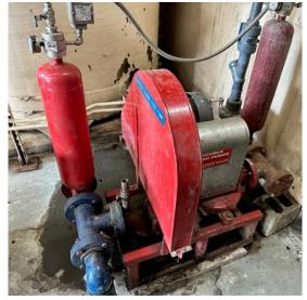
**Polymer System:** The polymer system does not have an indication of concentration. A batch of diluted polymer is sent to a 50-gallon tank. From there it is pumped to the floccuator at a ratio of the sludge flow.
