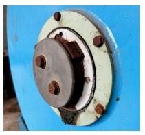
**Three-way valve:** The existing three-way valve does not work. It has been stuck in the dewatering position and does not turn. This causes problems with a proper startup. Sludge also leaks out of the supply tank, through the sludge pump and, because the valve is stuck in the dewatering position, into the channels.
