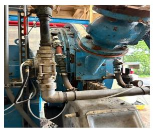
**Sludge Pump:** The facility has a double disc sludge pump and is in good condition. However, the sludge tank gravity feeds past the pump when it is in the off position.
