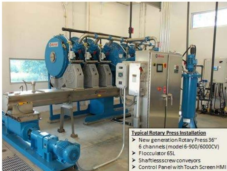
The filtrate passes through the screens as the flocculated sludge advances within the channel. The sludge continues to dewater as it travels around the channel, eventually forming a cake near the outlet side of the press. The frictional force of the slow moving screens, coupled with the controlled outlet restriction, results in the extrusion of a very dry cake.
