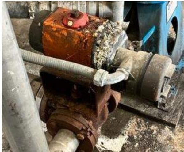
**Flocculator:** The flocculator seal shaft has been leaking for some time. It's hard to tell the extent of the damage.
