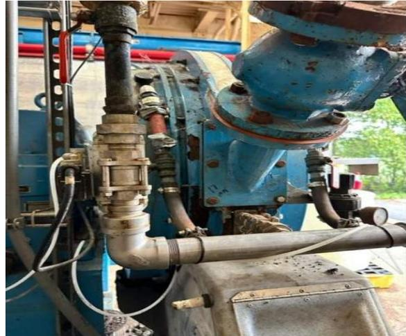
**Sludge Pump:** The facility has a double disc sludge pump and is in good condition. However, the sludge tank gravity feeds past the pump when it is in the off position.
