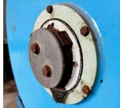
**Three-way valve:** The existing three-way valve does not work. It has been stuck in the dewatering position and does not turn. This causes problems with a proper startup. Sludge also leaks out of the supply tank, through the sludge pump and, because the valve is stuck in the dewatering position, into the channels.
