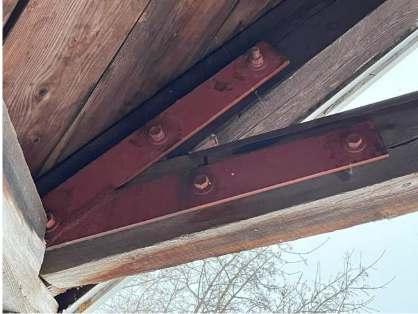
TRUSS HEEL JOINT CONNECTION
