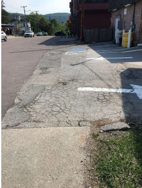
Figure 3: Gap in Sidewalk near Cumberland Farms
