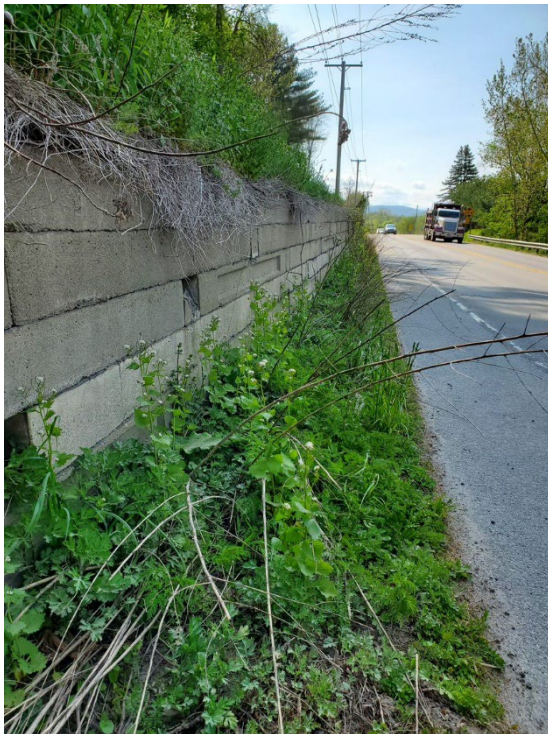
Figure 2: Retaining wall facing east.
