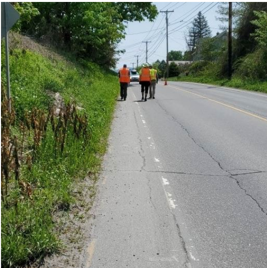
Figure 8: Embankments along US-2 heading into Richmond Village
