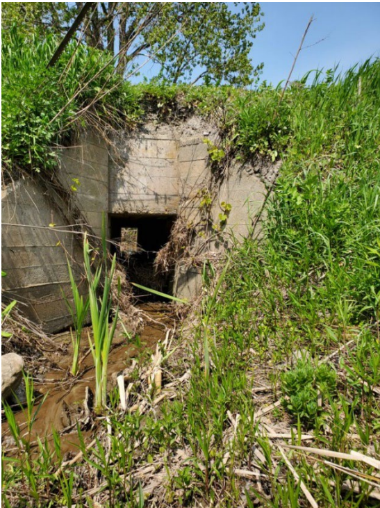
Figure 5: Inlet side of box culvert.
