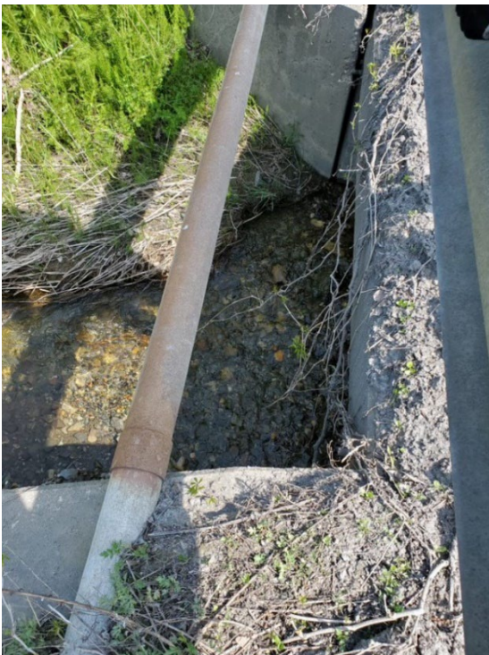
Figure 4: Eastbound (outlet) side of culvert.
