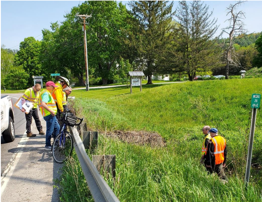
Looking westbound on US-2 towards the culvert.
