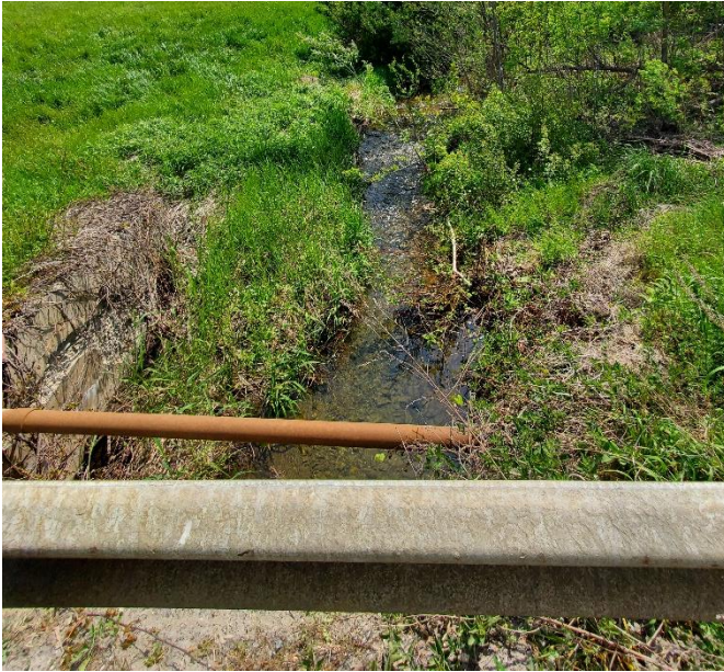
Upstream (left) and downstream (right) of culvert
