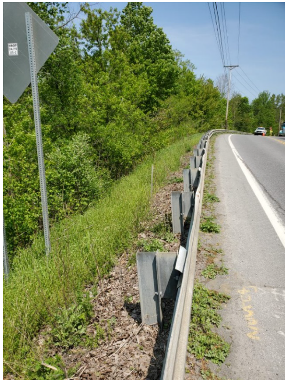
Figure 6: Embankment on US-2 facing West.
