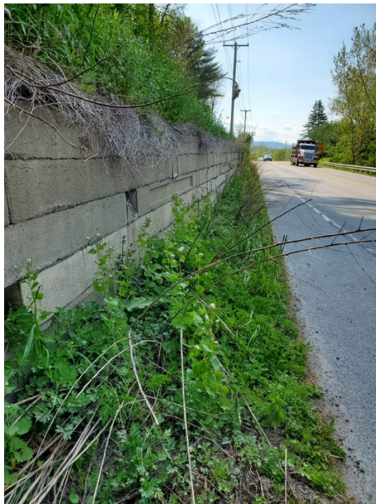
Figure 2 (Location 1): Retaining Wall facing East.
