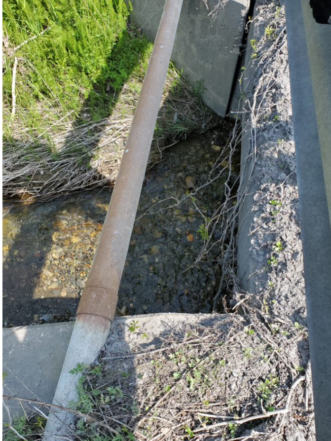
Figure 4 (Location 4/5): Eastbound (Outlet) side of Culvert
