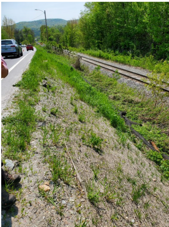
Figure 7: Embankment facing Eastbound along US-2
