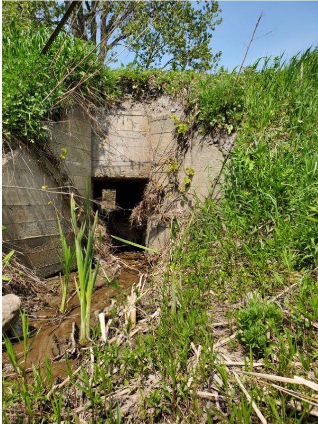
Figure 5: Inlet Side of Box Culvert
