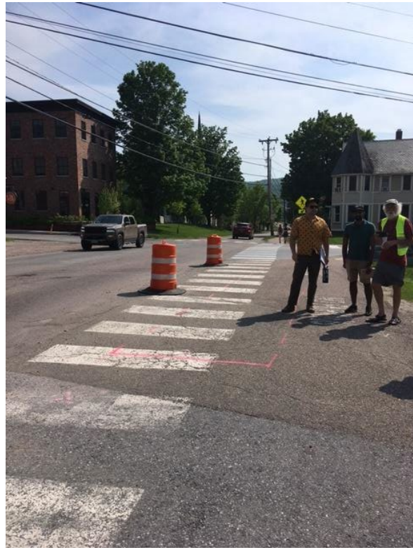
Missing Sidewalk next to Richmond Market
