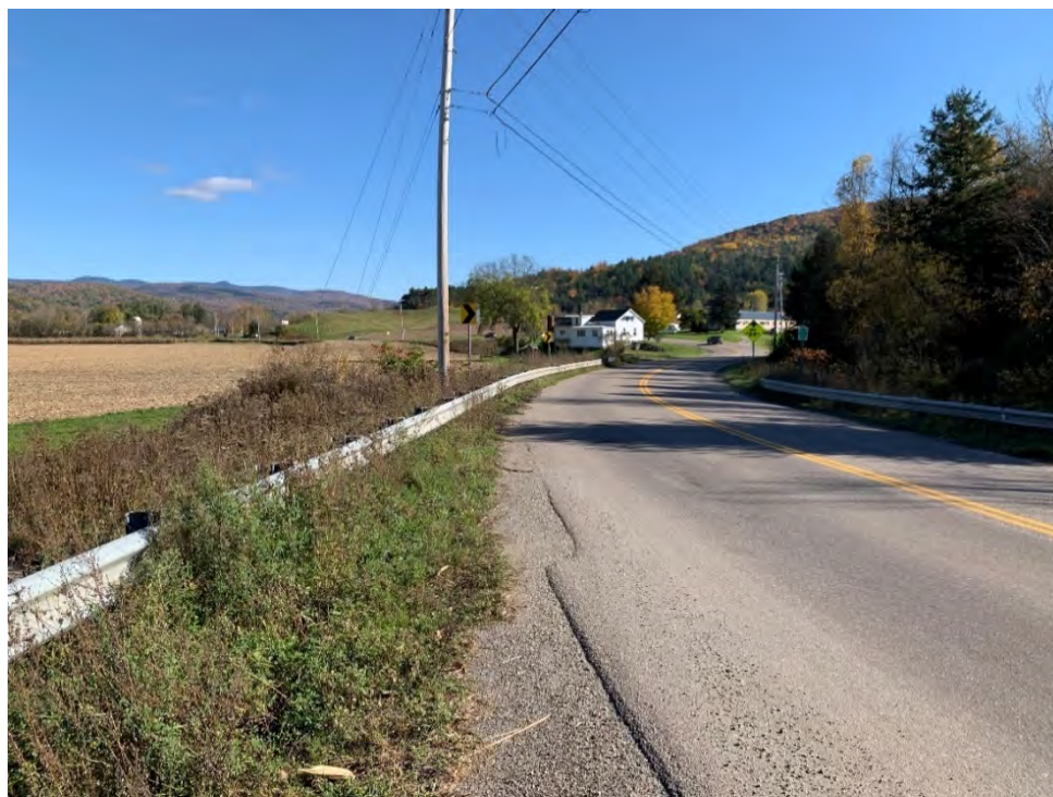
Figure 9 Huntington Road looking east
