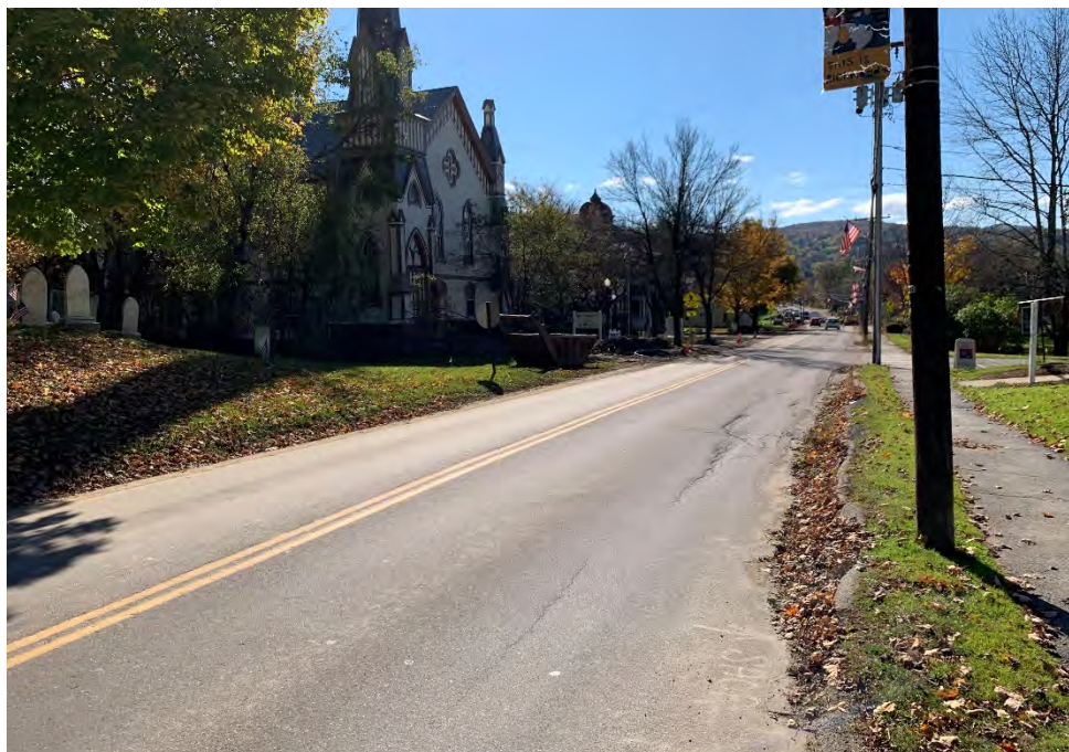
Figure 19 Bridge Street Existing Conditions - No-Action Alternative
