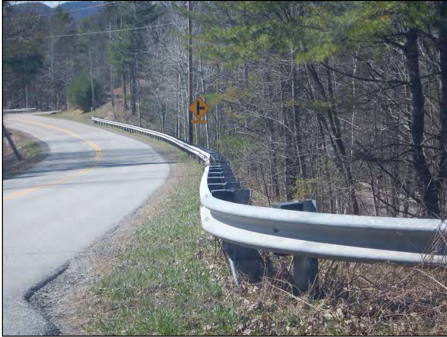
Photo 10. Photo shows the guide rail on the west side of Jericho Road. View is to the south.
