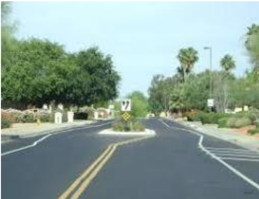
Figure 9 Typical Center Median
