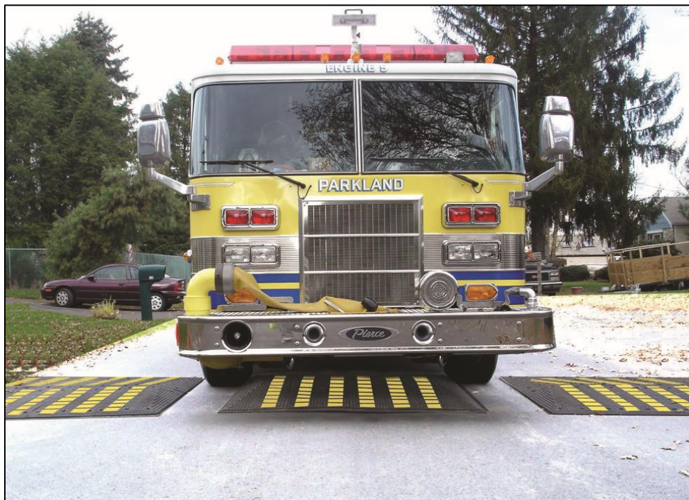
Figure 3 Typical Speed Cushion
