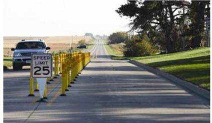
• A curb extension using paint and bollards:
