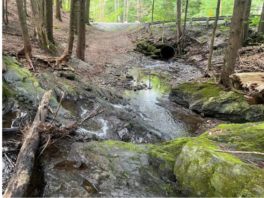
Figure 1. Photograph taken looking downstream at the Stage Road culvert inlet.
