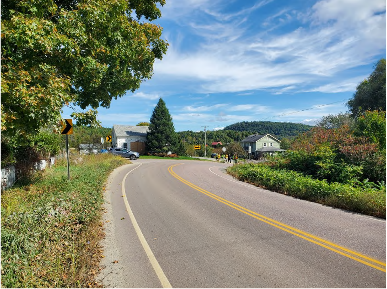
Figure 3: Hinesburg Road northbound approach at Fay's Corner
