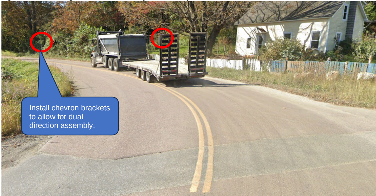
Figure 8: Hinesburg Road southbound just south of East Hill Road
