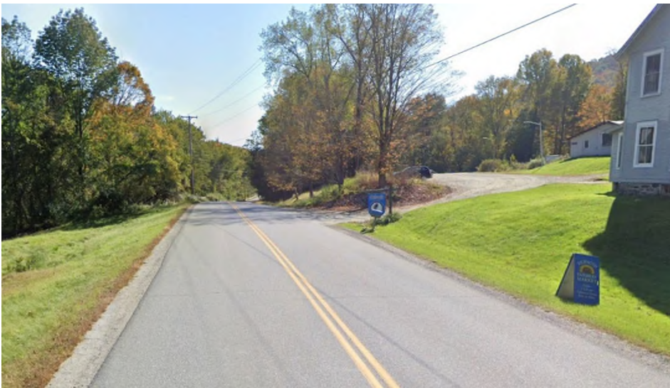
Figure 2: Looking east at the intersection of Cochran Ski Area driveway
