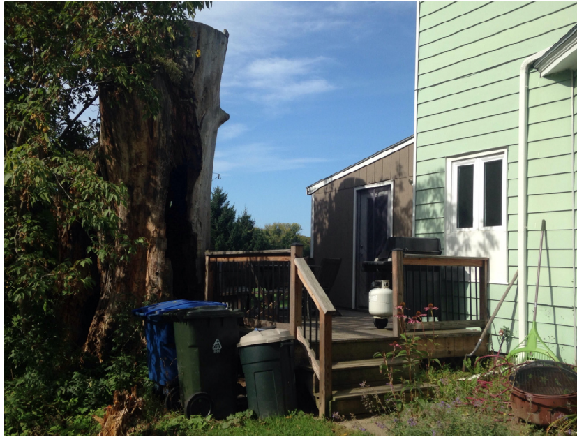
Easterly Side (side view) - Photo taken 9/20/17
