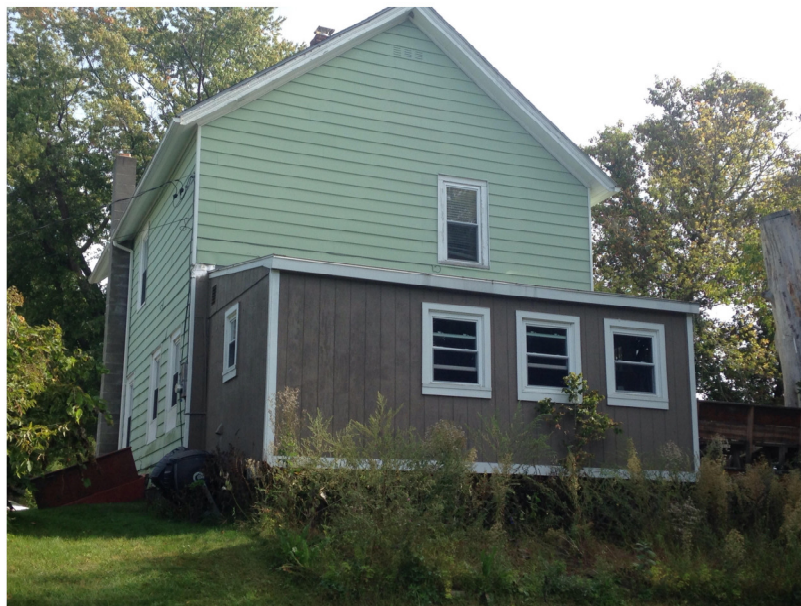
Southerly and Westerly View (rear and side view) - Photo taken 9/20/17
