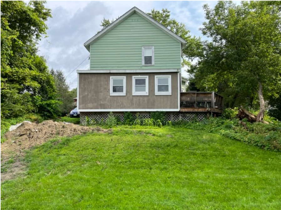
Picture 3: Rear (south) elevation. (Basement drain pipe discharge on left.)
