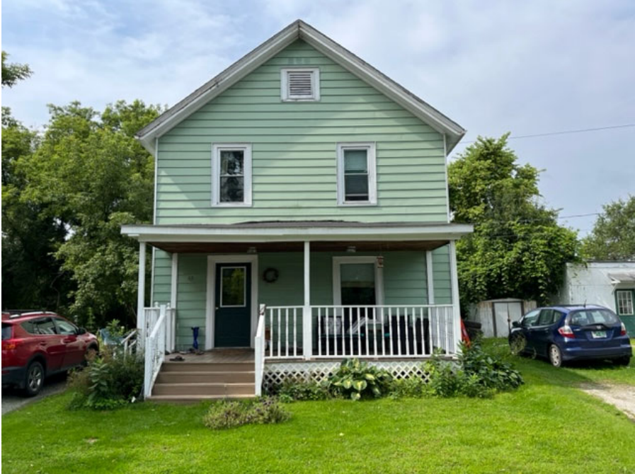
Picture 1: Front (north) elevation.
