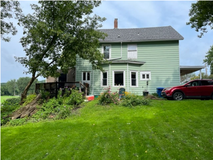
Picture 4: Left side (east) elevation.
