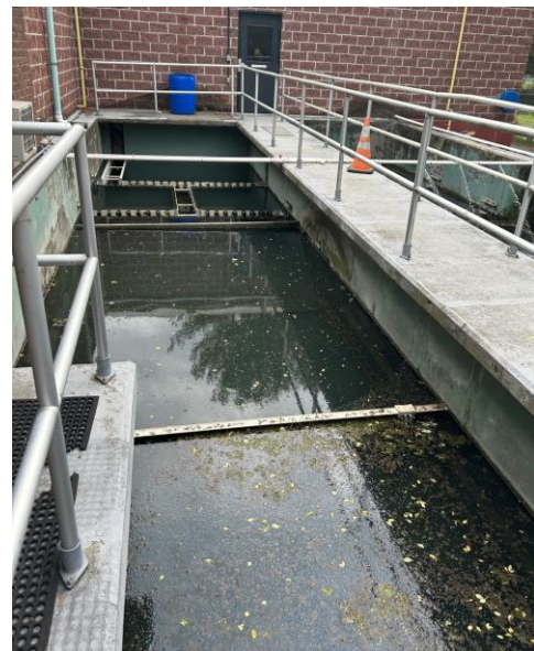
Figure 2-16 Secondary Clarifier
