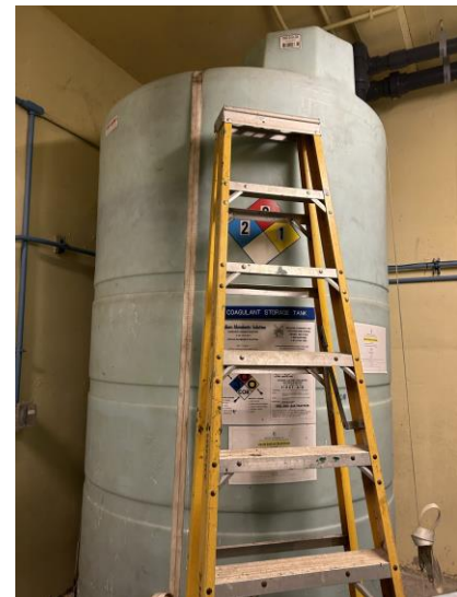
Figure 2-15 Sodium Aluminate Storage
