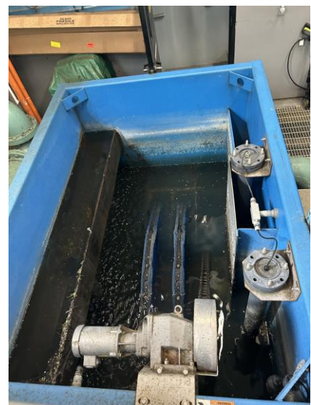
Figure 2-18 Filtration Tank
