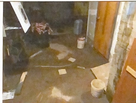
Town Center Basement Boiler & Elevator Room Door
