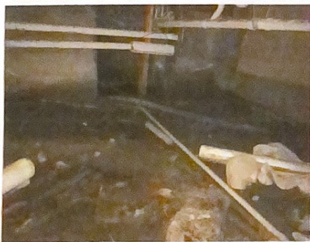
Town Center Basement and Crawl Space
