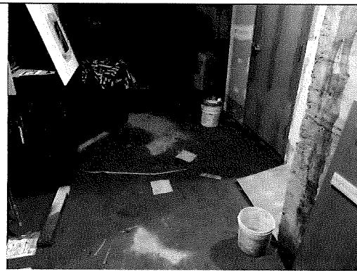
Town Center Basement Boiler & Elevator Room Door
