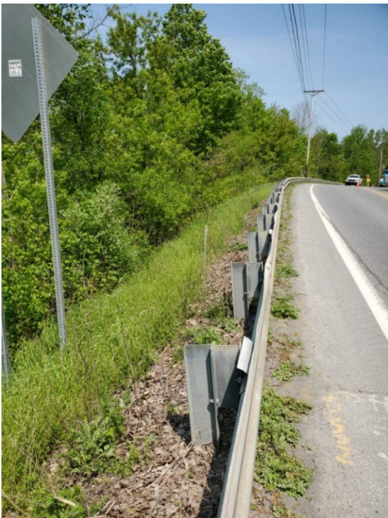
Figure 6: Embankment on US-2 facing west.
