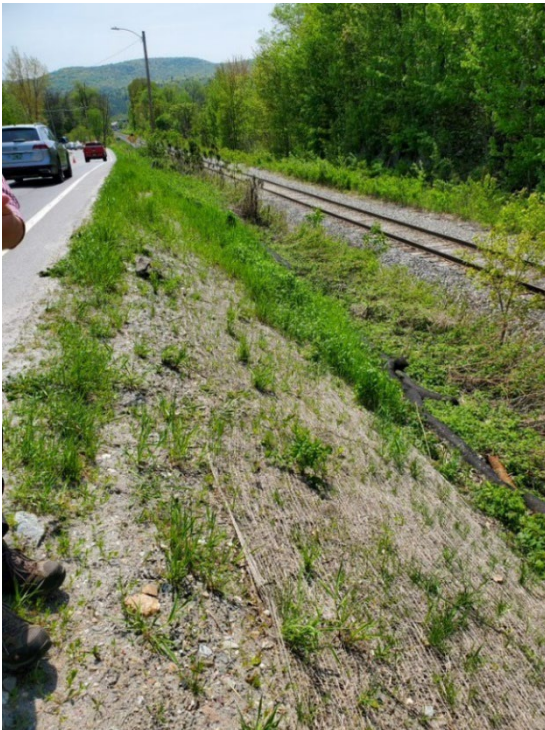
Figure 7: Embankment facing eastbound along US-2.
