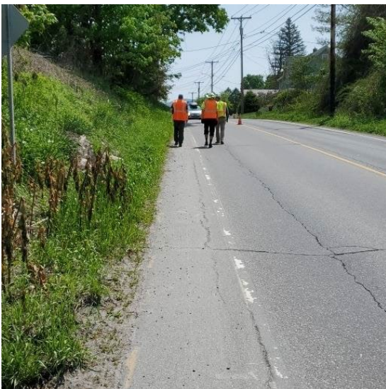
Figure 8: Embankments along US-2 heading into Richmond Village
