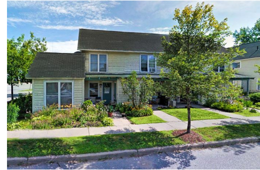
Richmond Village Housing- Borden St. Credit: Champlain Housing Trust
