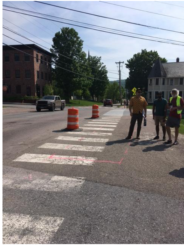
Missing Sidewalk next to Richmond Market
