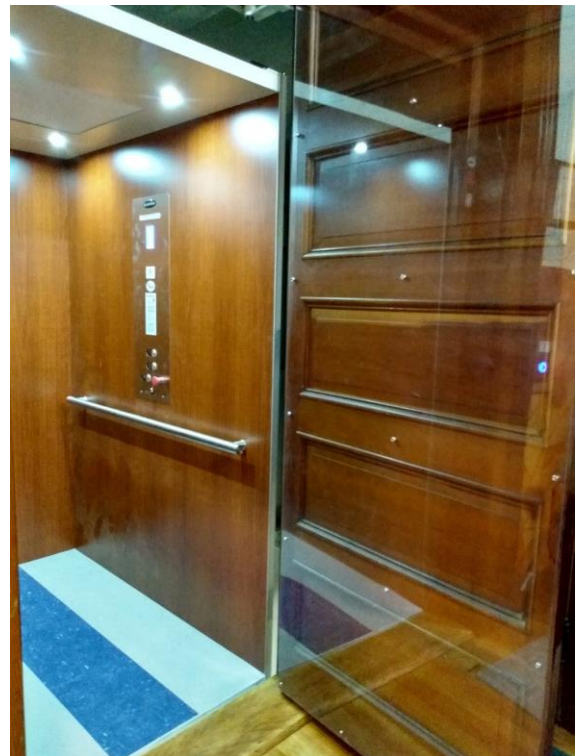
The vertical platform lift for accessibility used an existing door to minimize its visual impact on the historic interior.
