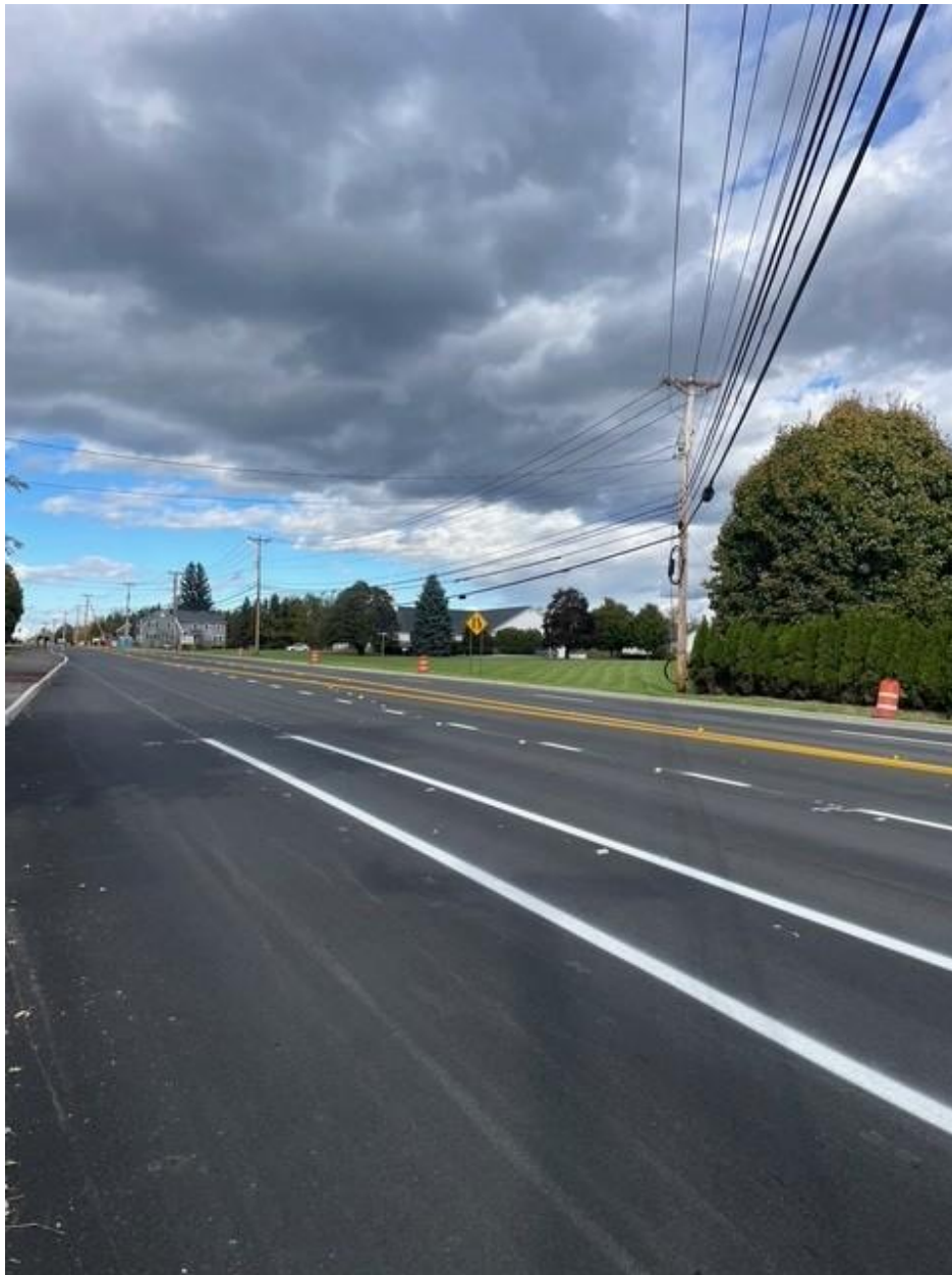
Crews install final line striping on VT 2A in Williston, VT.
