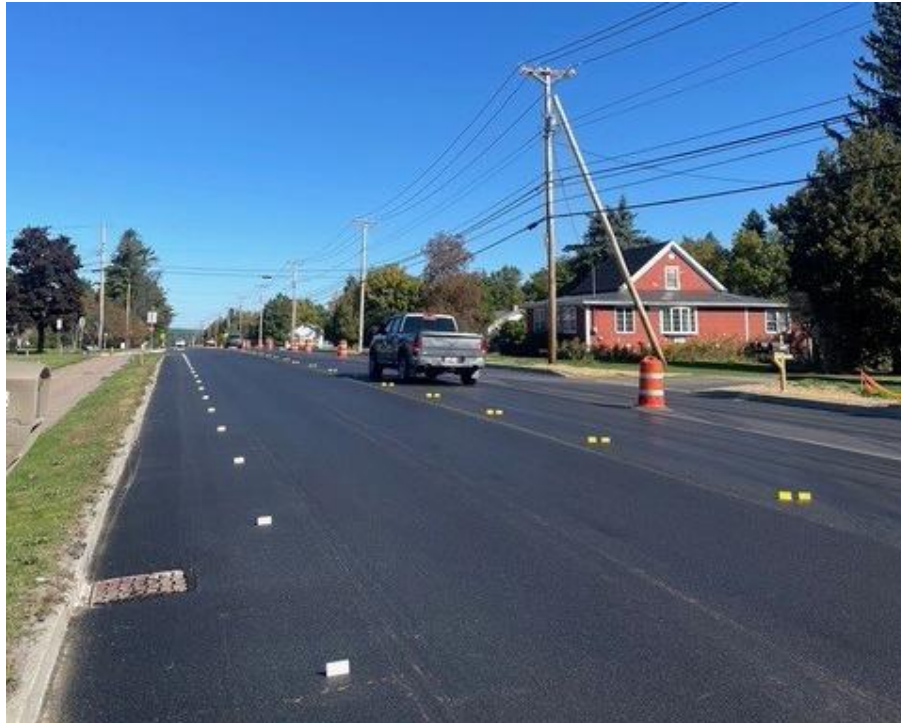
Crews pave the final wearing course of asphalt throughout the project limits in Williston, VT.
