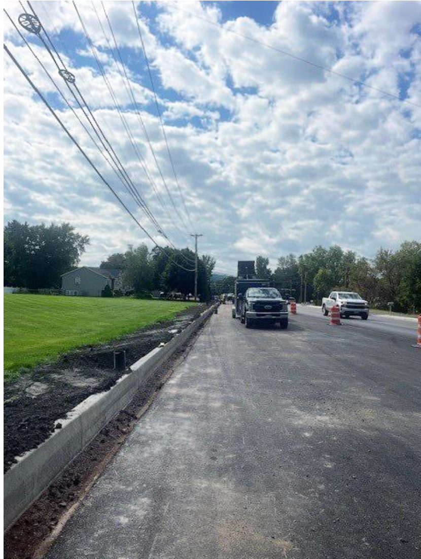
Crews place topsoil along VT 2A in Williston, VT.
