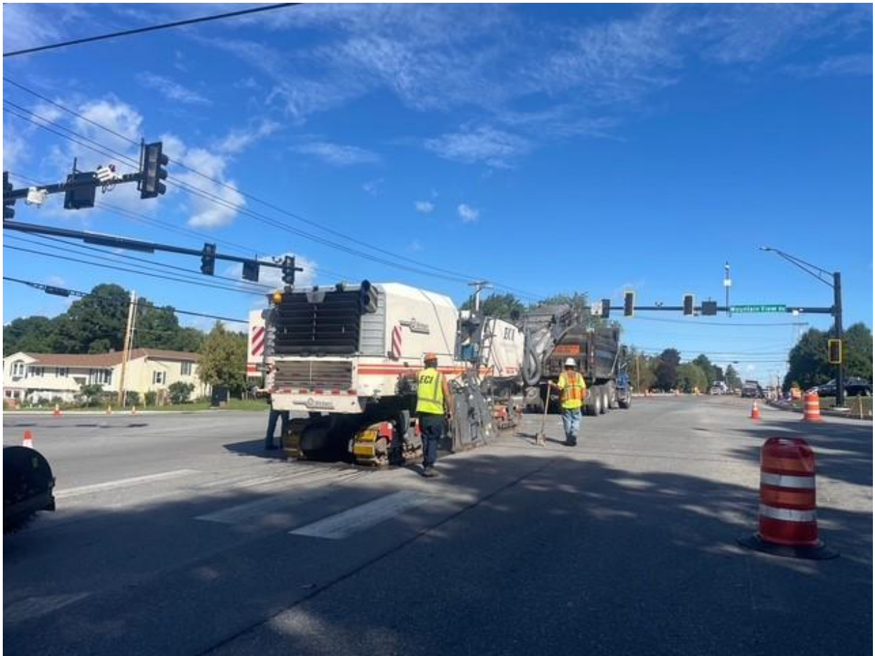
Crews mill the roadway within the VT 2A/Industrial Avenue/Mountain View Road intersection in Williston, VT.
