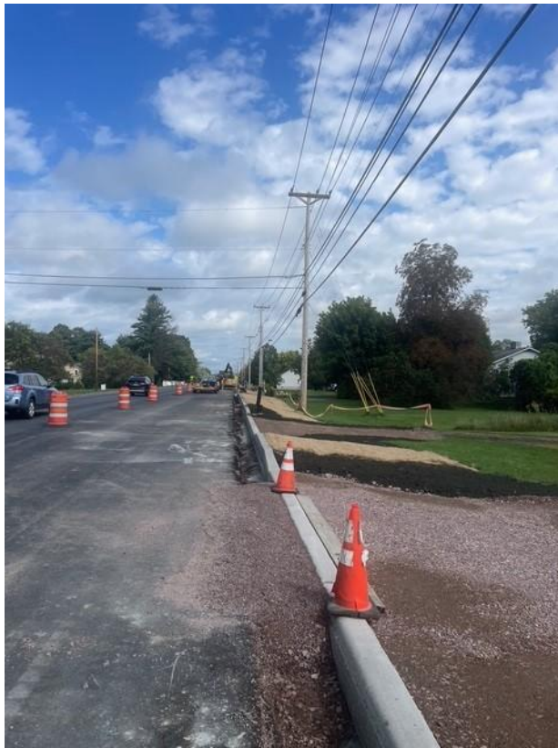
Crews place curb backing on the east side of VT 2A between Mountain View Road and just south of River Cove Road, including topsoil and temporary gravel driveway aprons.
