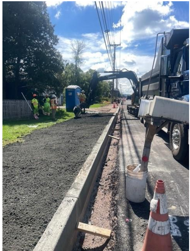
Crews place curb backing on the east side of VT 2A between Mountain View Road and just south of River Cove Road, including topsoil and temporary gravel driveway aprons.
