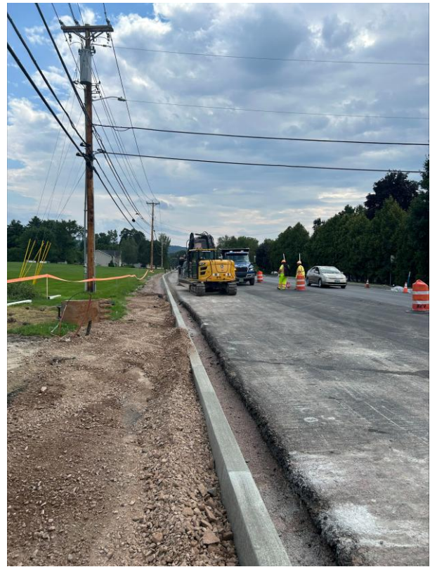
Crews install curb on the east side of VT 2A between Mountain View Road and just south of River Cove Road in Williston, VT.
