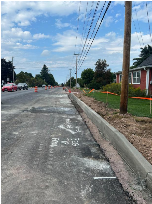
Crews install curb on the east side of VT 2A between Mountain View Road and just south of River Cove Road in Williston, VT.
