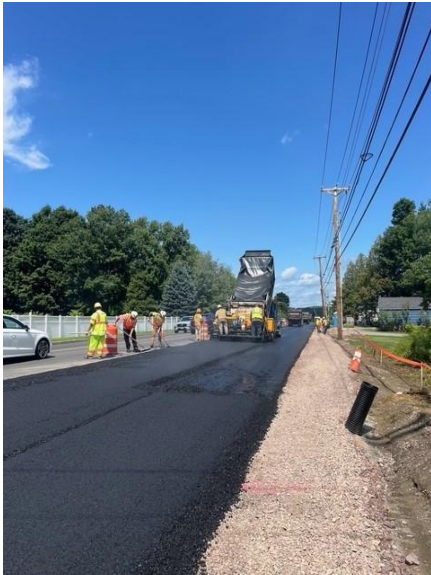
Crews pave the base layer of asphalt along the newly widened east side of VT 2A in Williston, VT.
