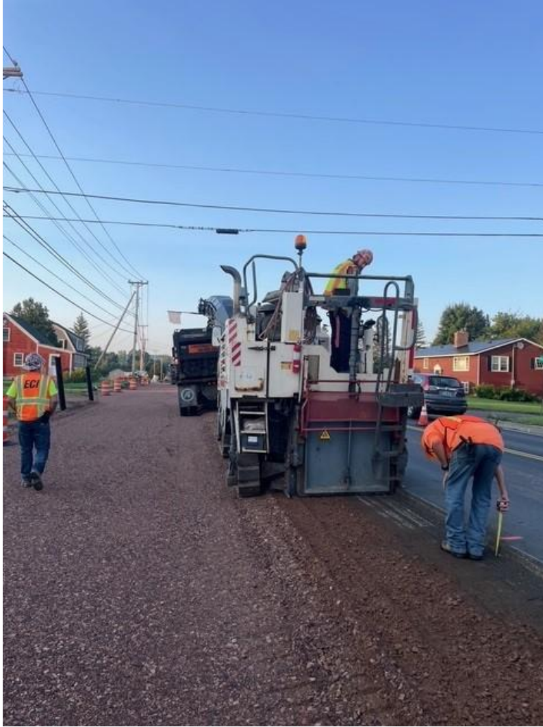
Crews conduct milling on the east side of VT 2A near Hillside Drive in Williston, VT.
