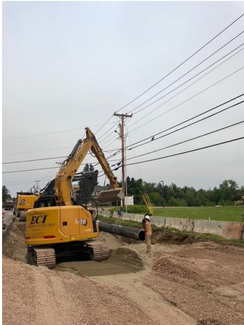
Crews install drainage infrastructure along the east side of VT 2A in Williston, VT.
