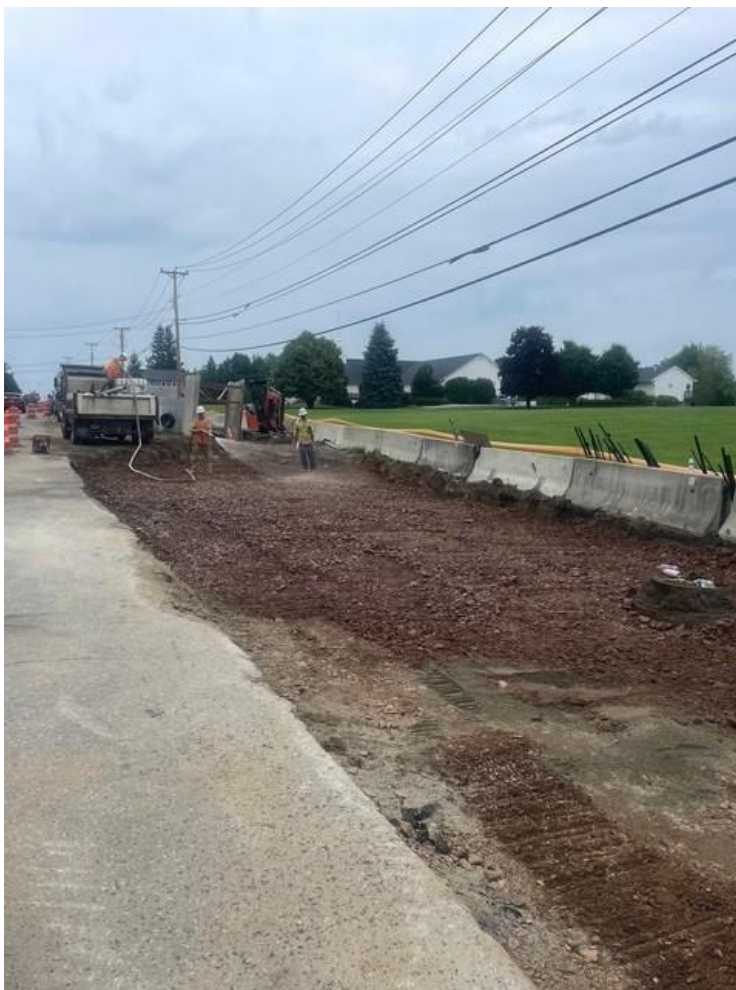
After conducting roadway widening along the east side of VT 2A in Williston, VT, crews backfill the area with gravel and spray for dust control.
