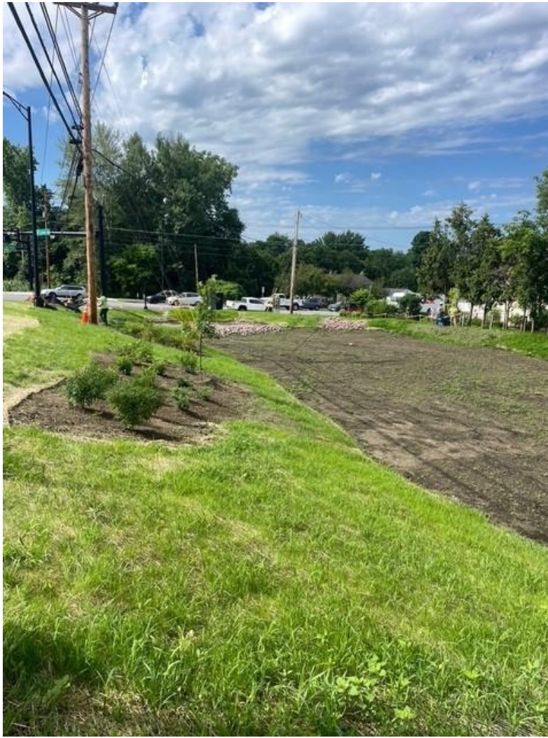
Plants are placed at the new bioretention pond on the corner of VT 2A and Industrial Avenue in Williston, VT.
