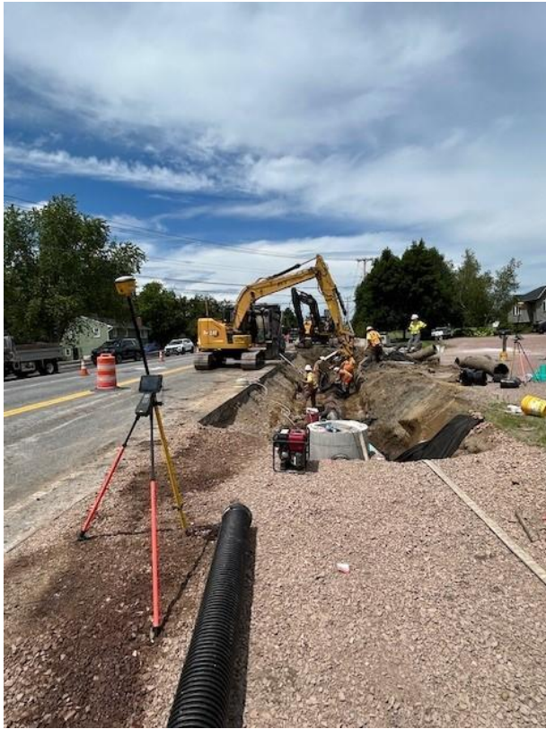
Roadway widening and drainage infrastructure installation take place along the east side of VT 2A between Mountain View Road and Sharon Drive in Williston, VT.
