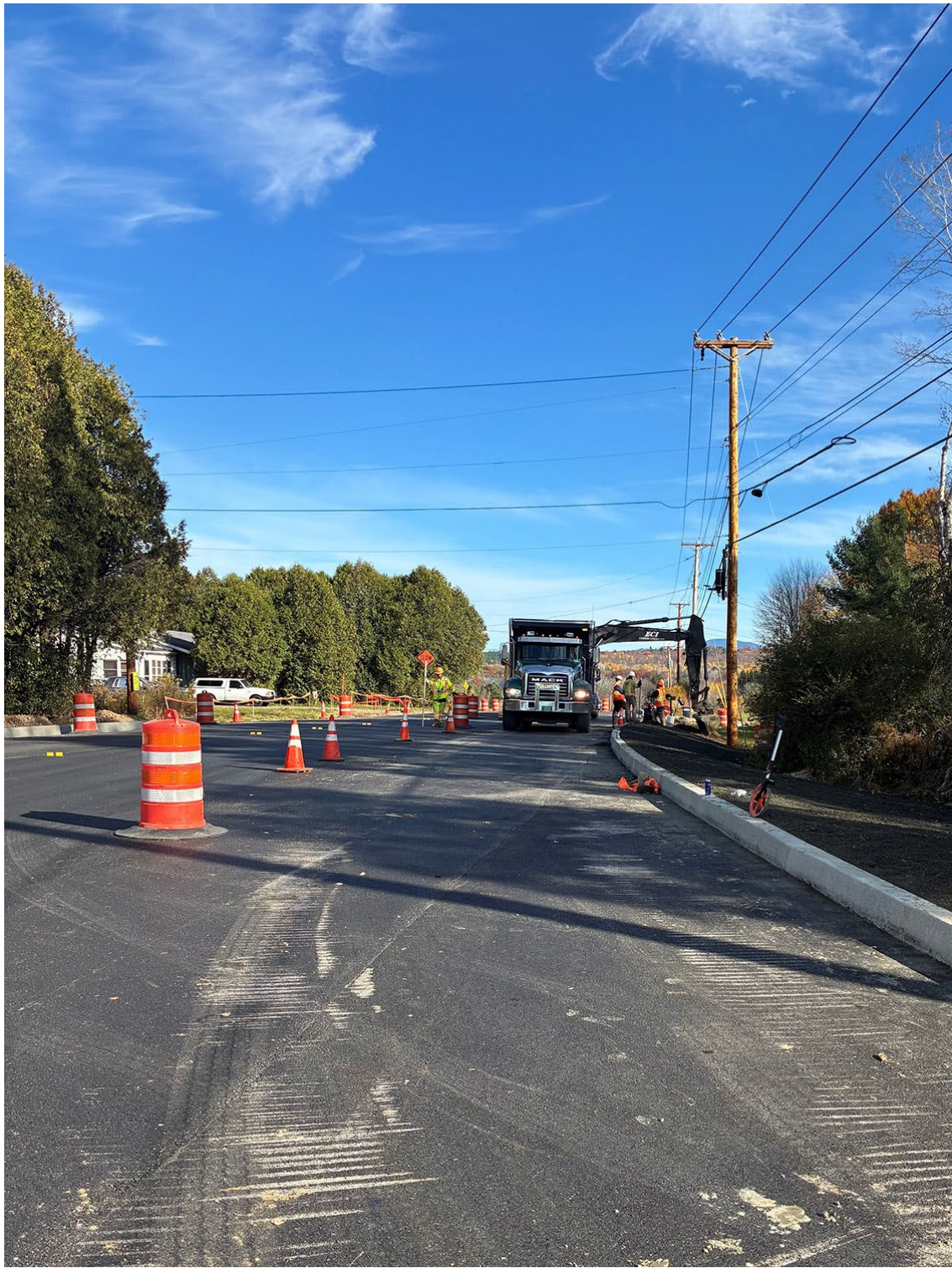
Crews place topsoil along the south side of Mountain View Road in Williston, VT.
