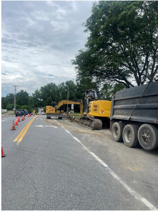
Crews widen the roadway and install drainage along VT 2A southbound between Meadowrun Road and Industrial Avenue in Williston, VT.
