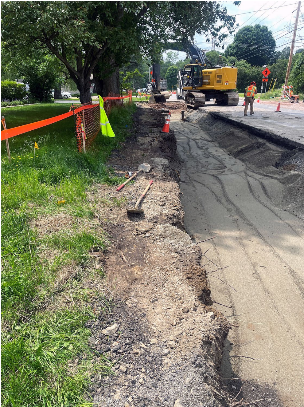
Crews conduct roadway widening along the south side of Industrial Avenue between Gail Terrace and VT 2A in Williston, VT.
