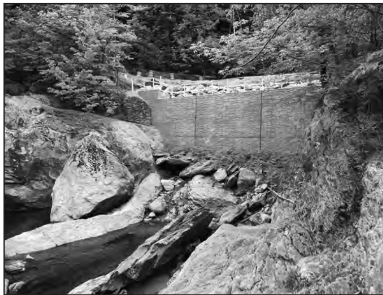
Repairs to the retaining wall at Huntington Gorge.
