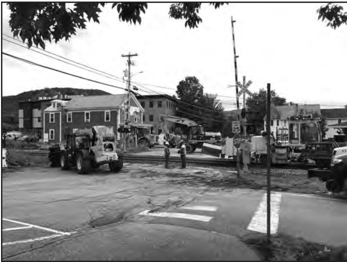
Repair of Railroad Crossing on Bridge Street.
