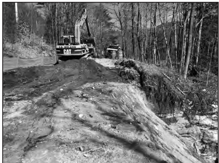
Work on the reconstruction of Dugway Road.
