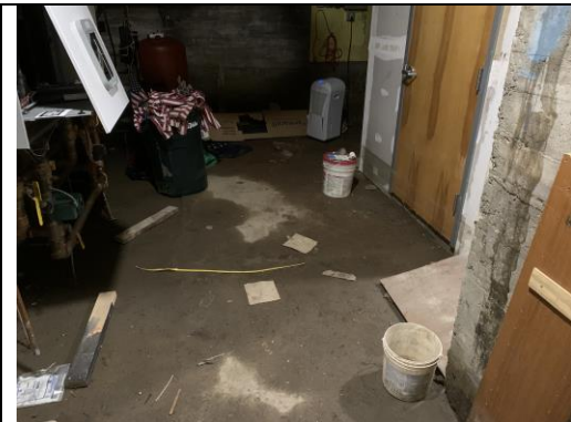
Town Center Basement Boiler & Elevator Room Door
