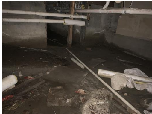
Town Center Basement and Crawl Space
