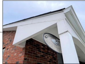
REMOVE EXISTING ROOF RETURNS ON CUSTOMER ENTRANCE PORCH. EXTEND SOFFIT AND ADD NEW ROOF RETURN FLUSH WITH WALL, SAME HEIGHT.
