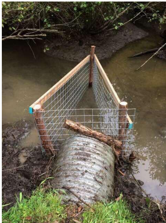
Triangle fences can work at small culverts and where space is limited.
