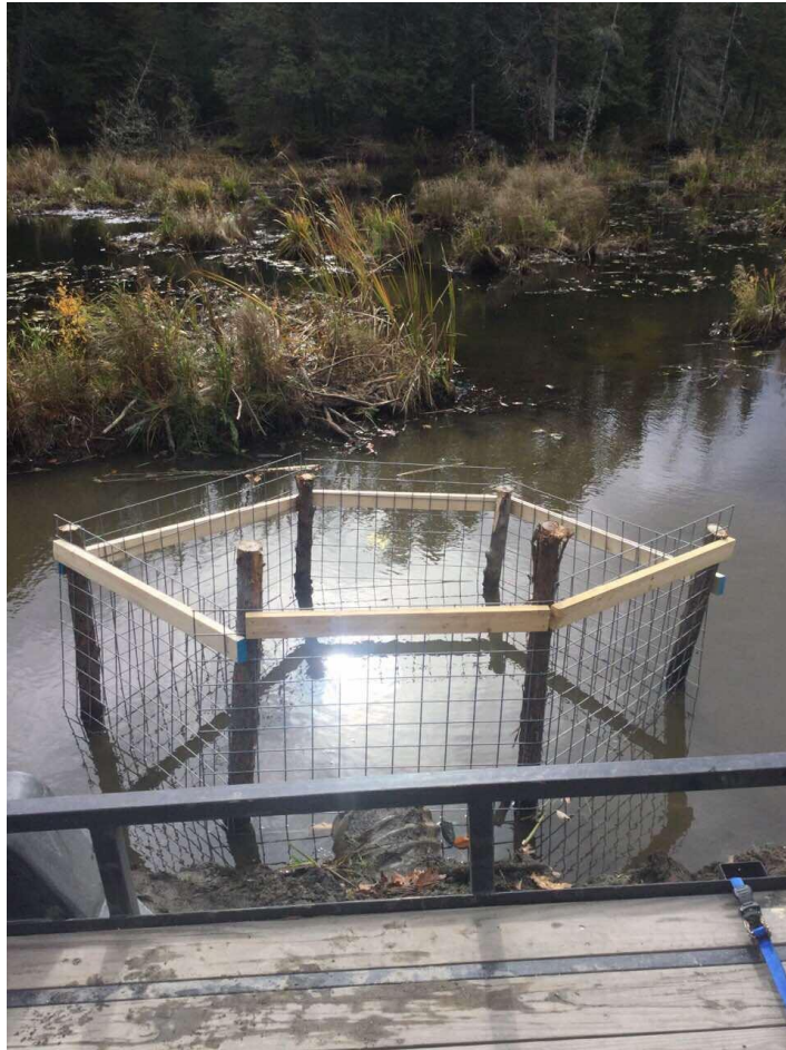
Diamond shaped fences create sharp angles that seem to deter beavers
