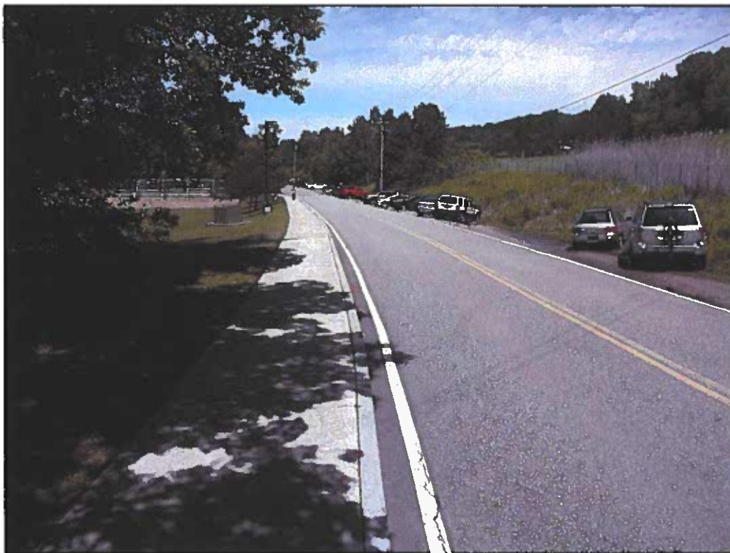
Photo 9. Entrance to Camel's Hump Middle School. Note cut bank on the right and sidewalk with embankment on the left. View to the northwest.
