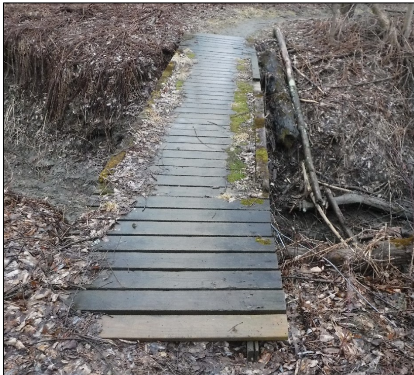
Image of one of the bridges to be replaced
