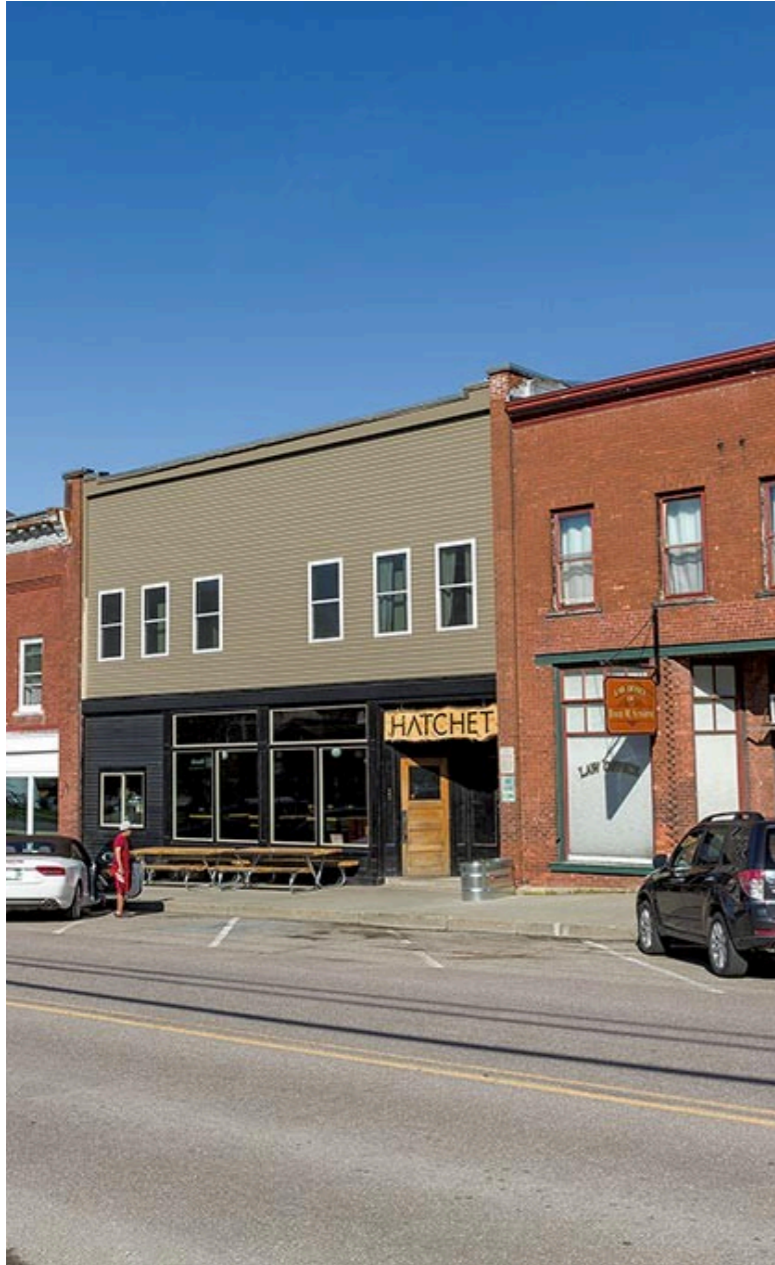
Bridge Street, Richmond Village
