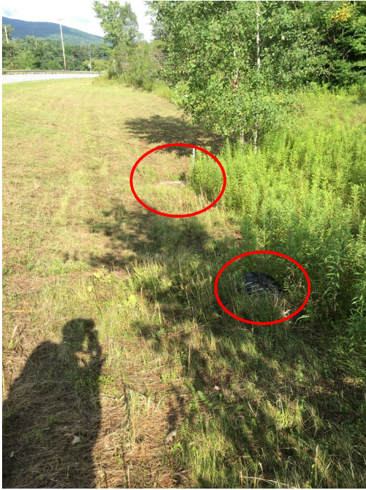
Drainage structures near entrance
