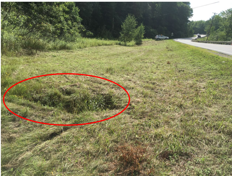
Another large hole – approx. 5 ft. x 3 ft. wide and 1 ft. deep
