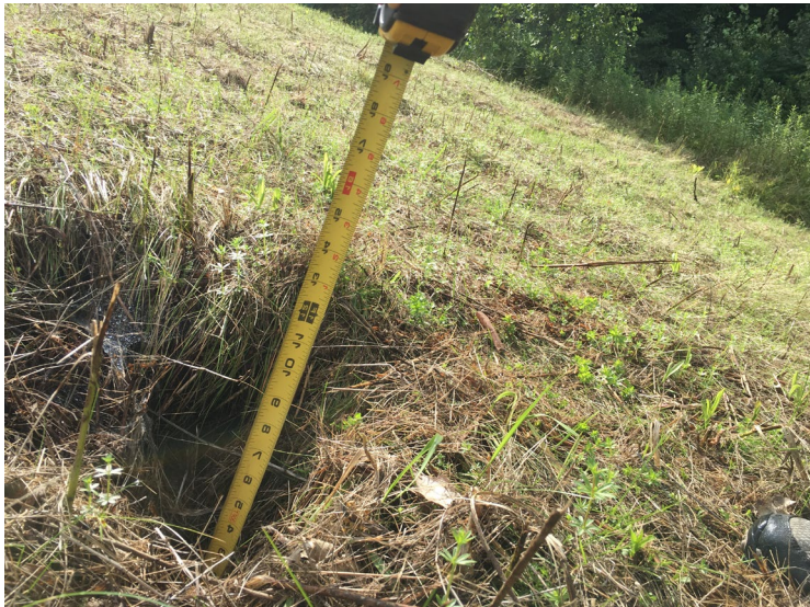
Hole near entrance (one of several)
