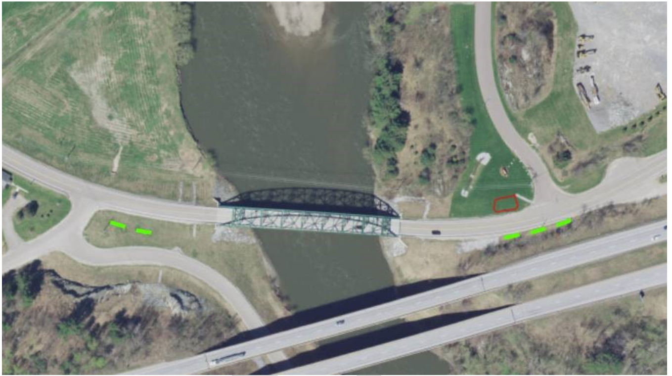
Figure 7 Stormwater Infrastructure near Bridge #24
