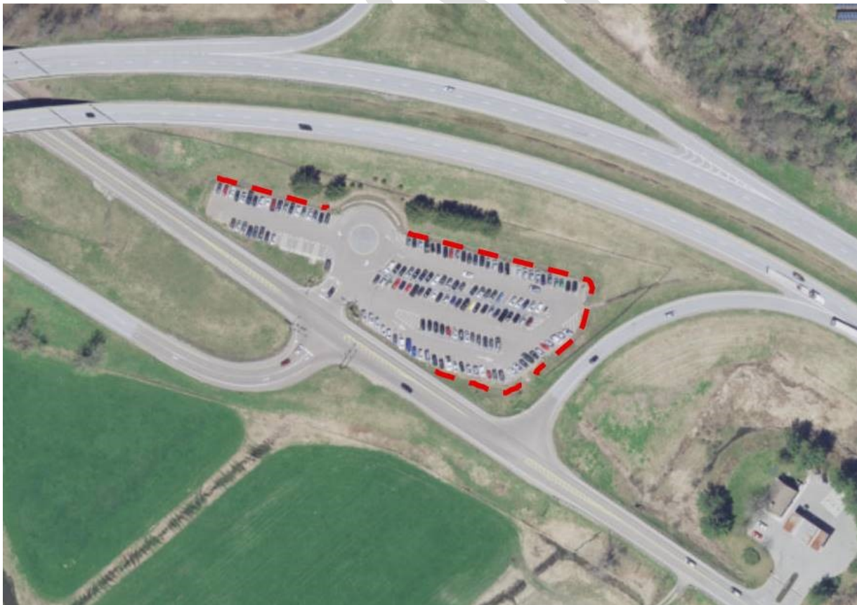
Figure 8 Stormwater Infrastructure Near Park & Ride
