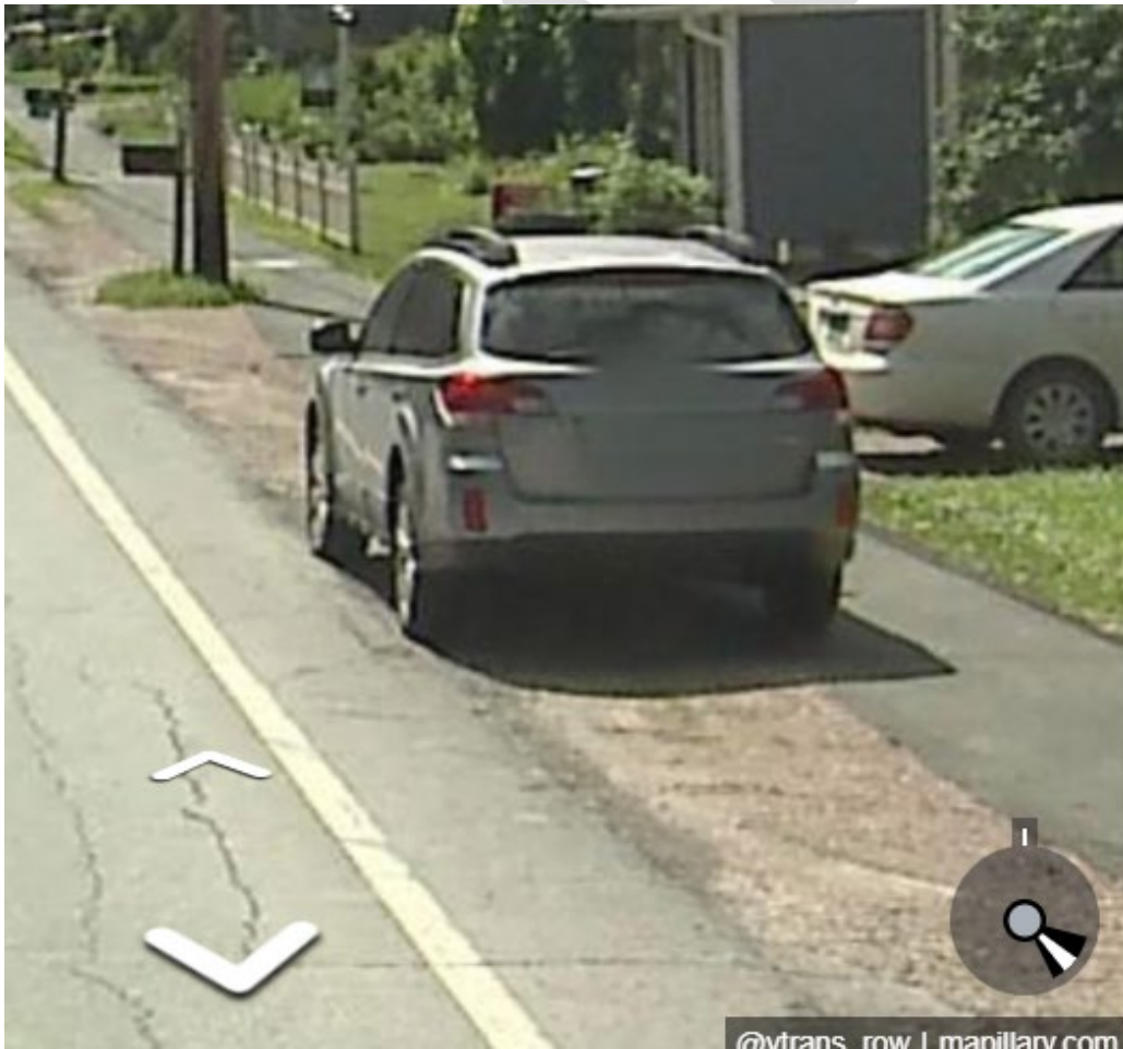
Figure 6 Richmond Parking - East Side of Intersection - Eastbound
