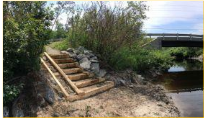
Figure 3. Example of stairs with boat ramp shortly after installation.
