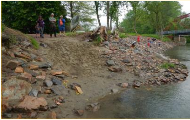
Figure 2: Steep slope from the river to the Green. People use the rip rap to fish despite the uneven footing.
