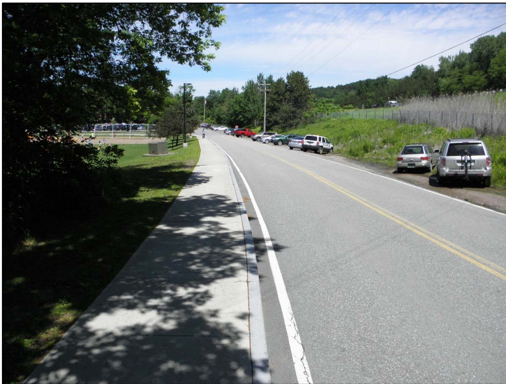
Photo 1. Entrance to Camel's Hump Middle School. Note cut bank on the right and sidewalk with embankment on the left. View to the northwest.
