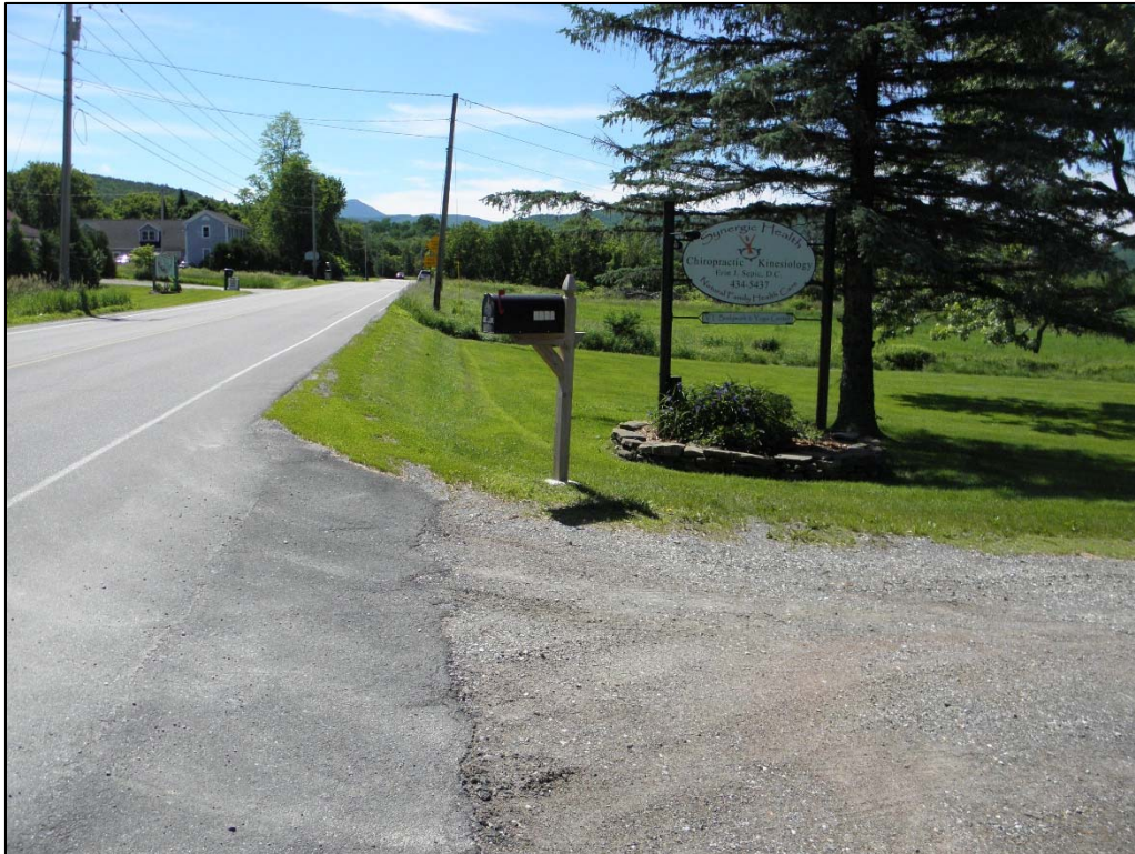
Photo 5. Terrace area adjacent to the Winooski flood plain on both sides of Route 2. Note low embankment in the foreground that increases in height in the background. View to the southeast.
