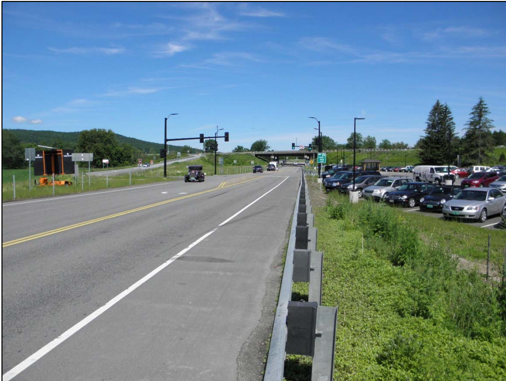
Photo 7. Disturbance of I-89 and associated park and ride lot. View to the northwest.
